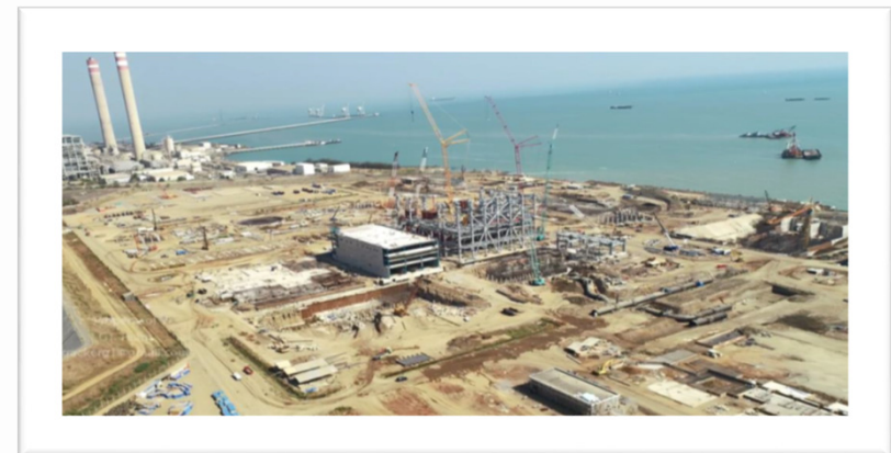
Photo: PLTU Jawa-4 (Tanjung Jati 5&6), September 2018
