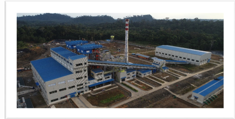
Photo: PLTU PAMA-1, September 2018
