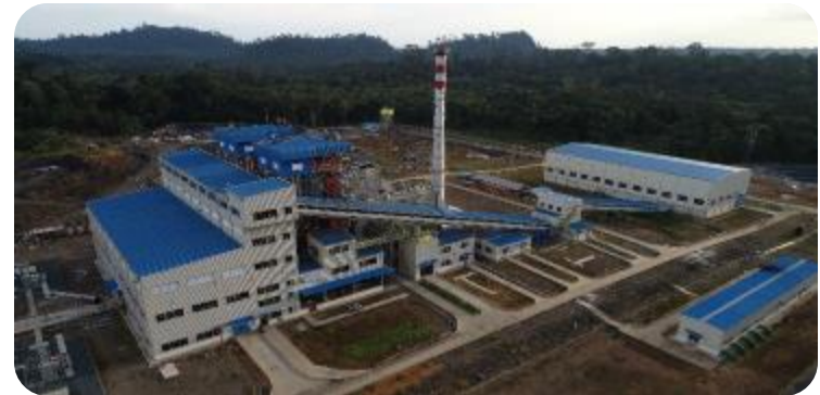
Photo: PLTU PAMA-1, September 2018
